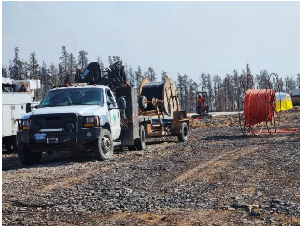
Northwestel technicians splice in several kilometres of new fibre last summer in the aftermath of massive wildfire activity in the South Slave region of the N.W.T. (Submitted by Northwestel)
